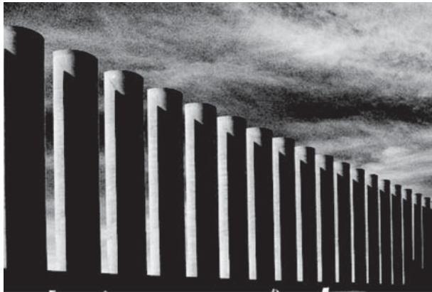
Fig. 7. Windscreen Calandkanaal – The Port of Rotterdam (The Netherlands)
