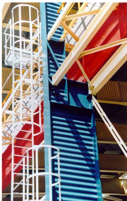
Fig. 3. Crane way column
