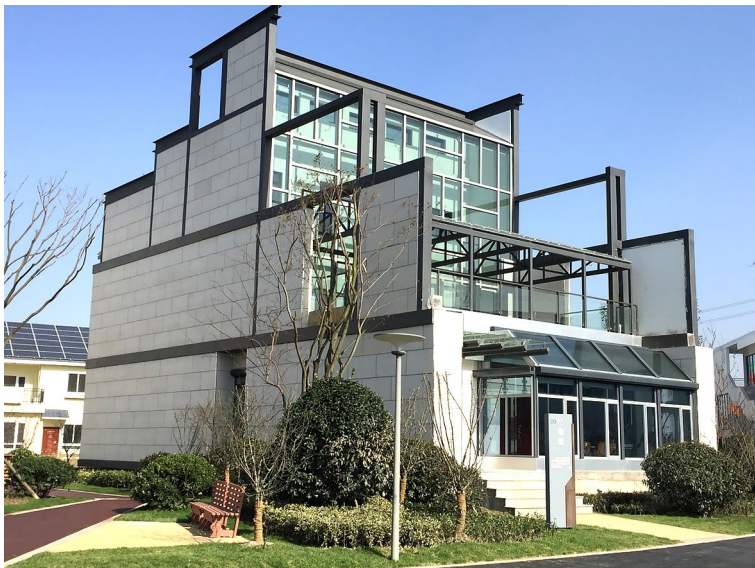
Figure 3. Yi Hui Tang building
