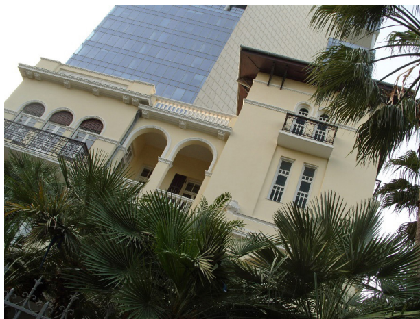
Figure 3. Example of an Eclectic Style building in the White City (source: the authors)
